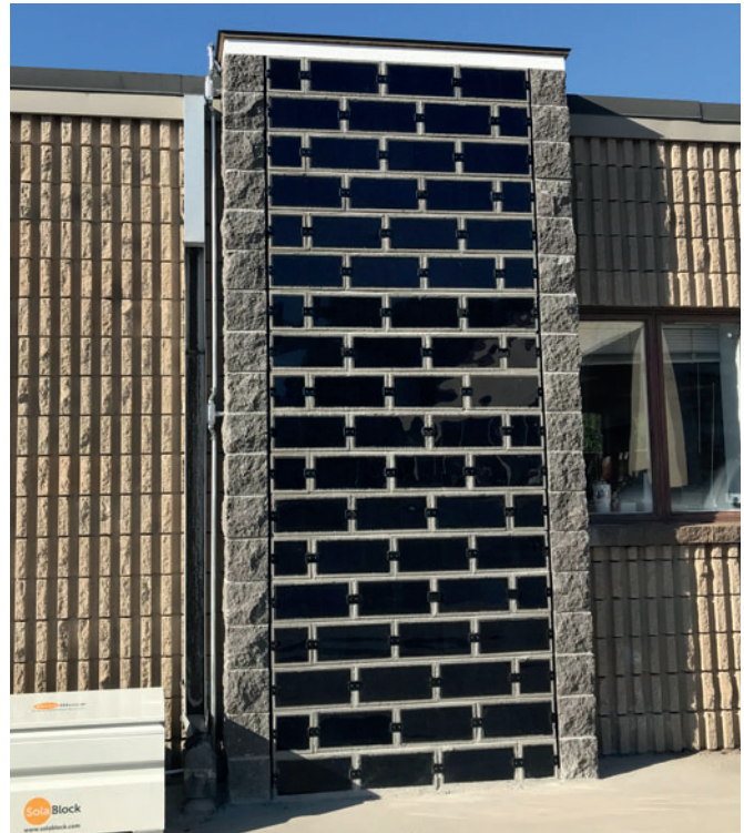
During the late summer 2019 installation of a demonstration solar wall on location, the solar SMUs attracted plenty of attention.
